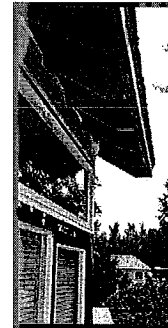
Open eaves, vents not screened (6 pts)
